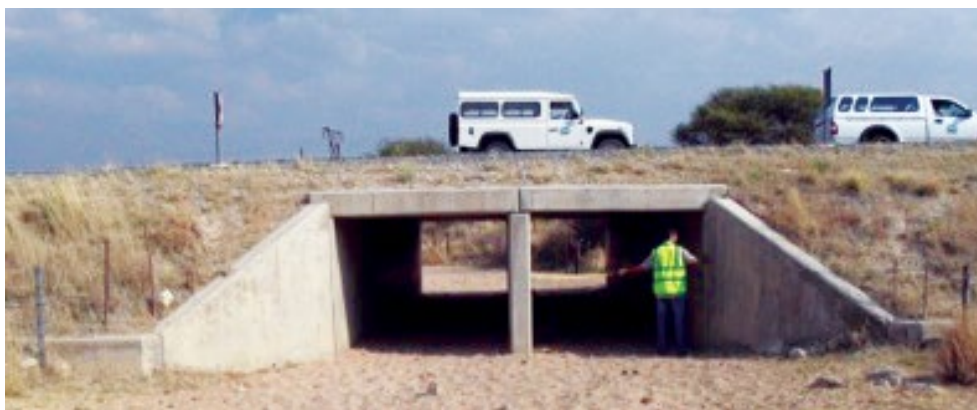
Figure 6: Culvert Dimensions Measurements
